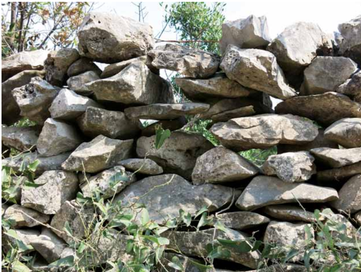
Injula gomila / Mur simple / Single drystone fence pile
