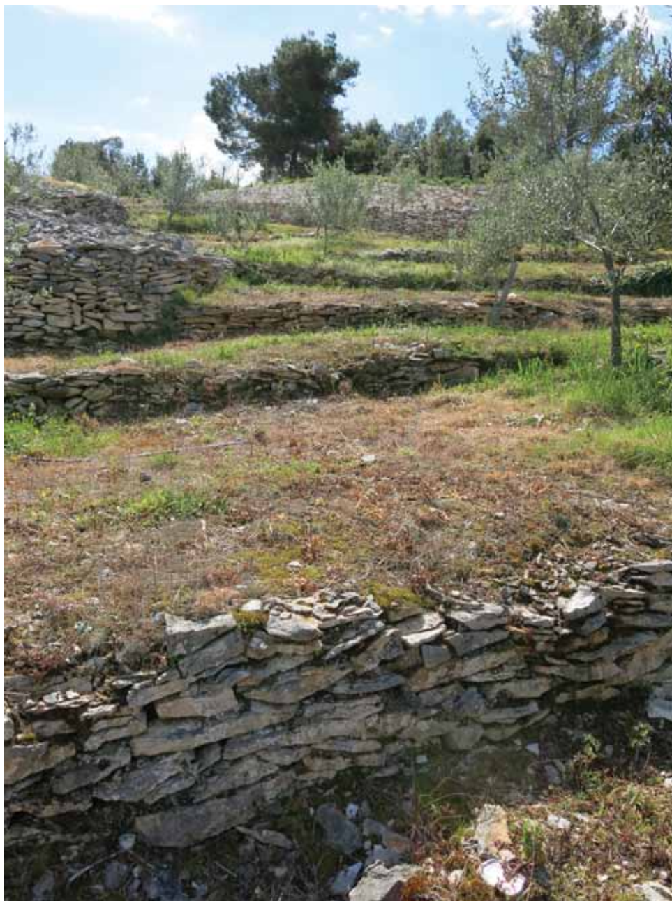
Podzidi (pristave) / Murs de soutènement (transversaux) / Drystone retaining walls ("pristave")
