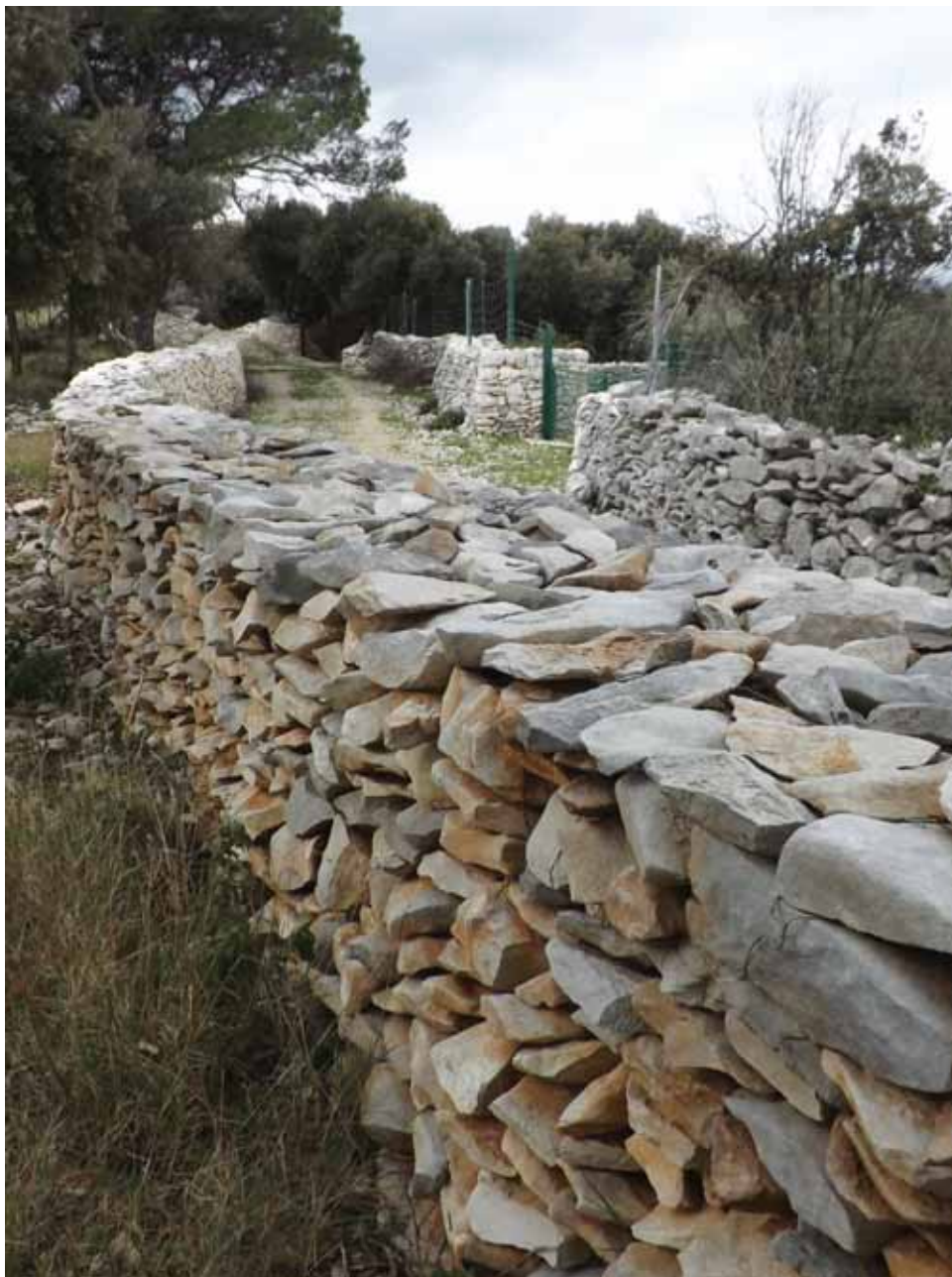
Dupla gomila pokrivena "plankaštrima" / Double mur couvert de grosses pierres plates / Double drystone fence pile covered with "plankaštri"
